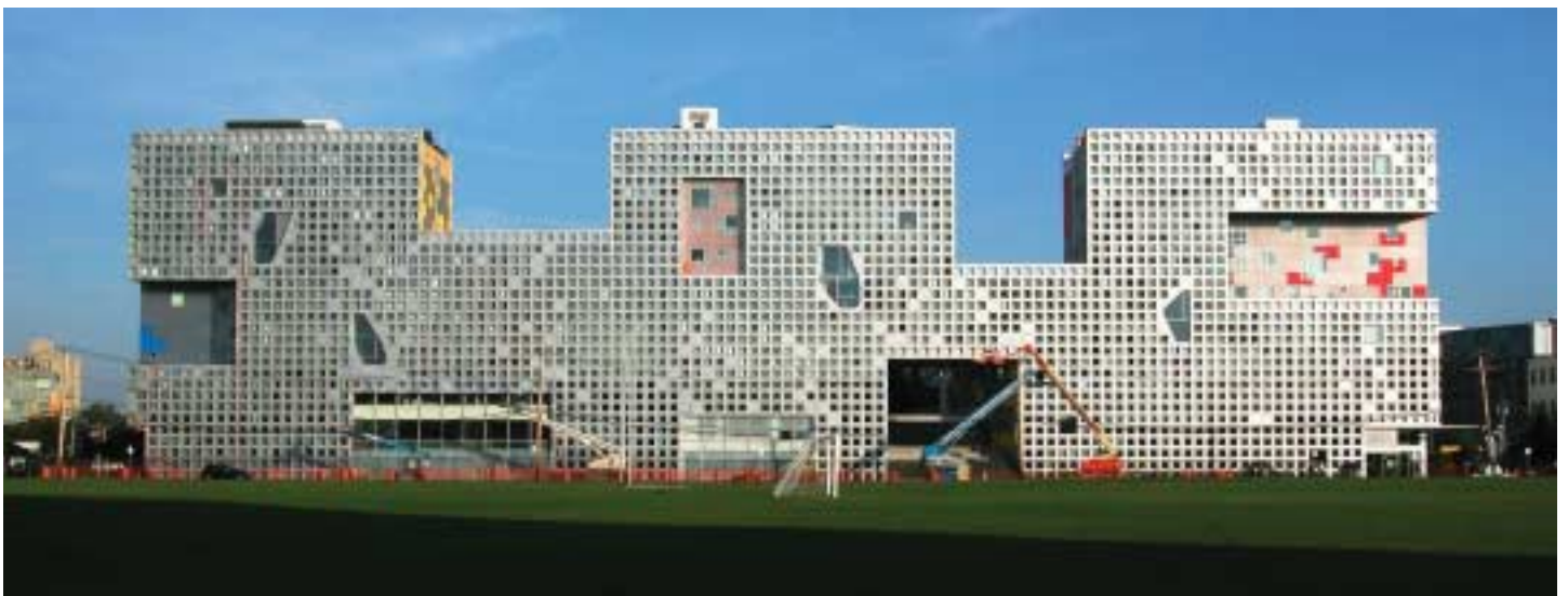
4. South façade of Simmons Hall under construction.
